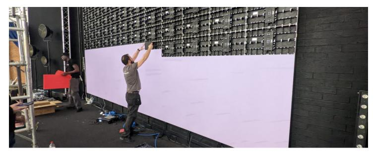
LED technology offered numerous advantages over the previous projection-based system. LED screens were significantly brighter, allowing for optimal visibility even in high ambient lighting conditions during live performances.
